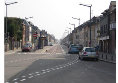
Figure 22.44. A virtual busway stop located in the middle of the roadway. *Andre Frieslaar.*
