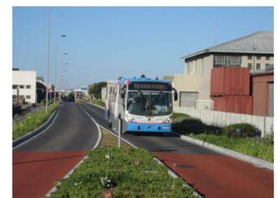
Figure 23.12. Section of colored friction course with ultrathin asphalt on Cape Town's MyCITI system. Aimee Gauthier
