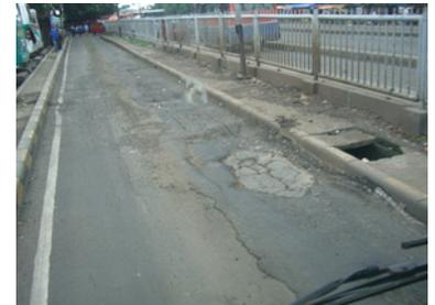
Figure 23.9. Transjakarta, in Jakarta, Indonesia, initially used only asphalt and suffered from major problems of the roadway sinking and deteriorating at the stations, so the roadbed at the stations was repaved using concrete. ITDP
