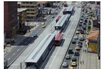
Figure 7.15. The use of multiple sub-stops, in this case three in each direction, has been one of the principal reasons Bogotá is able to achieve very high customer capacities. Photo Akiris.
