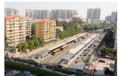
Figure 7.14. The use of multiple sub-stops and passing lanes helps minimize vehicle congestion in Guangzhou, China. Photo ITDP.
