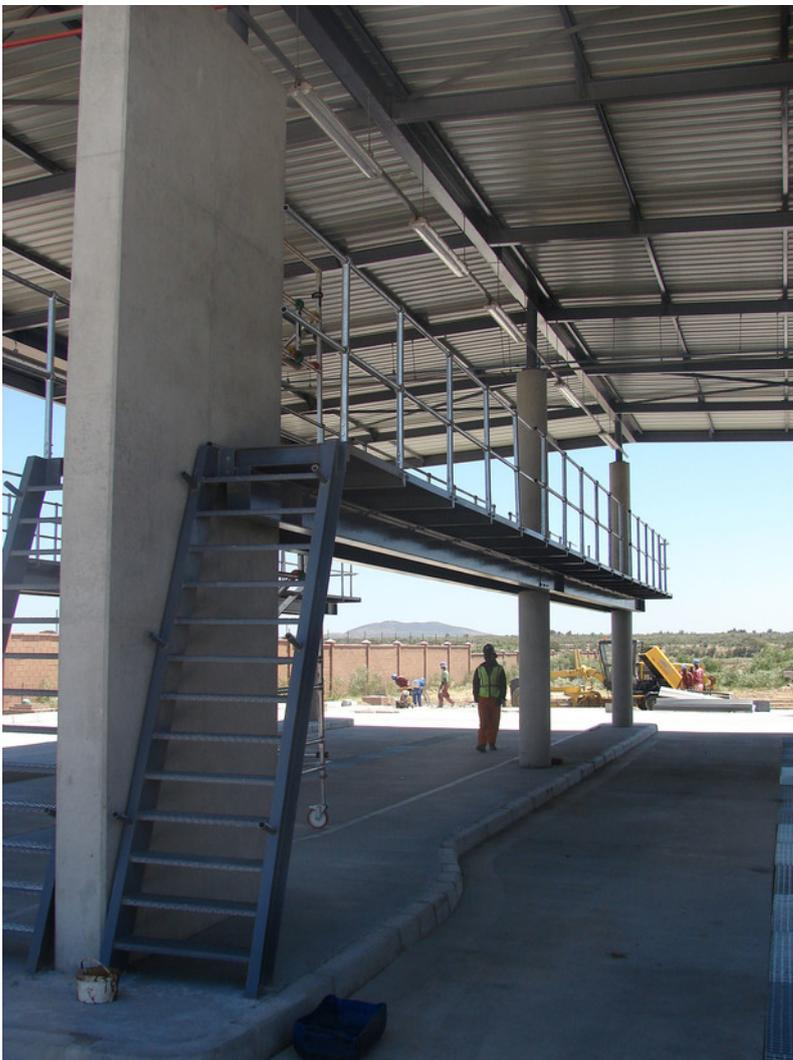
Figure 26.9. Stairs and a catwalk give access to the vehicle roof for washing purposes. *Andre Friestaar.*
