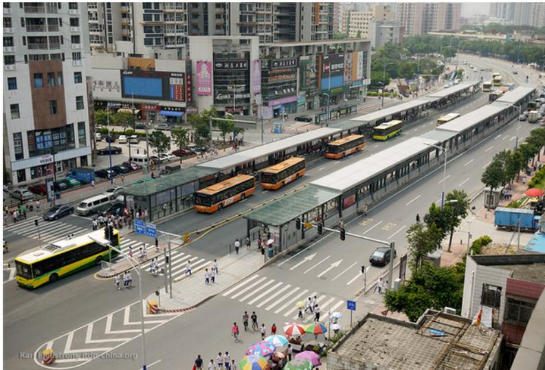
Figure 25.13. Dongpu BRT station in Guangzhou shows the station divisions including the access and arrival areas, the entrance area including the space for fare collection, and the three sub-stops, which can be identified by the different roof material and variation in elevation. At each sub-stop, multiple docking bays are seen and the station includes passing lanes. Between sub-stops is space for buses to pull into or out of the station around other buses already docked. Karl Fjellstrom.
