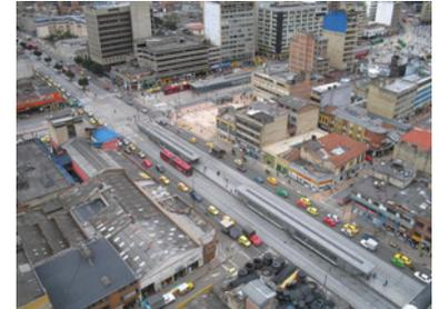
Figure 6.8. The use of multiple sub-stops and docking bays with passing lanes in Bogotá helps minimize vehicle congestion. Oscar Diaz and Por el País que Queremos (PPQ).
