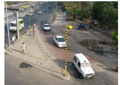
Figure 29.27. A raised crosswalk on the Delhi, India, busway helps reduce the speed of left-turning vehicles. *Chris Kost*
