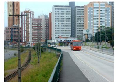
Figure 22.25. In this city-center location Curitiba, Brazil, is able to segregate the busway to the side of an existing railway. ITDP.
