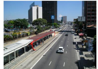
Figure 29.47. In São Paulo, this mid-block station is served by a pedestrian overpass, but does not have physical separation to keep customers from crossing travel lanes to access buses. *Michael King*
