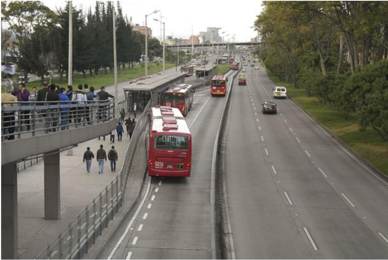
Figure 22.54. An interchange station in Bogotá, with a closed environment between the two trunk platforms. *ITDP*.
