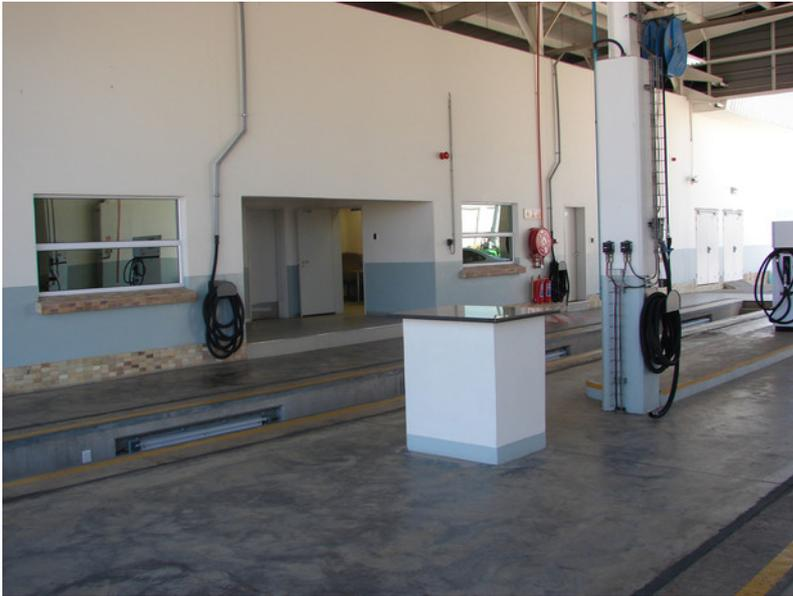
Figure 26.12. A pit beneath the work area allows technical staff to inspect (and service) the underside of the vehicle. *Andre Frieslaar.*
