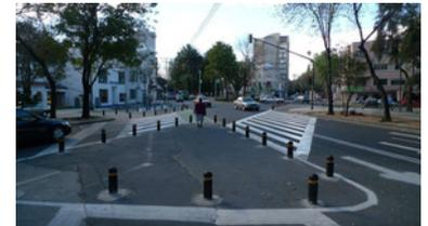
Figure 29.6. A redesigned intersection in Mexico City. The medians were extended into the intersection to reduce turning speeds and provide more pedestrian refuge areas, and crosswalks were brought into line with actual observed pedestrian movement. ITDP
