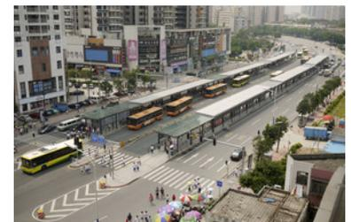
Figure 24.49. Dongpu BRT station in Guangzhou (see layout at Figure 24.45) provides at-grade station access at both ends, combined with mixed-traffic U-turns. Karl Fjellstrom.
