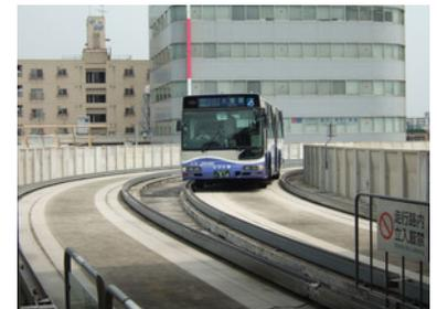
Figure 22.27. Nagoya, Japan's elevated BRT line utilizes a mechanical guidance system to reduce the required roadway width. *Lloyd Wright.*
