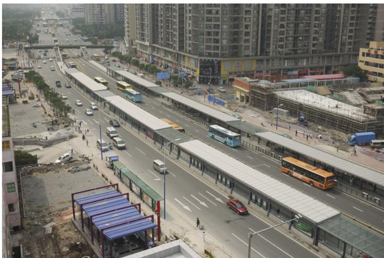
Figure 22.60. A multiple sub-stop, split, side-aligned station in Guangzhou, China. *ITDP.*
