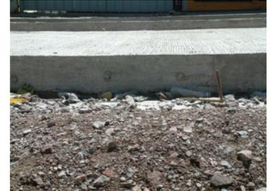
Figure 23.7. Reinforced concrete, as in this example from the construction of the Quito Central Norte line, has much greater longevity than asphalt. Lloyd Wright
