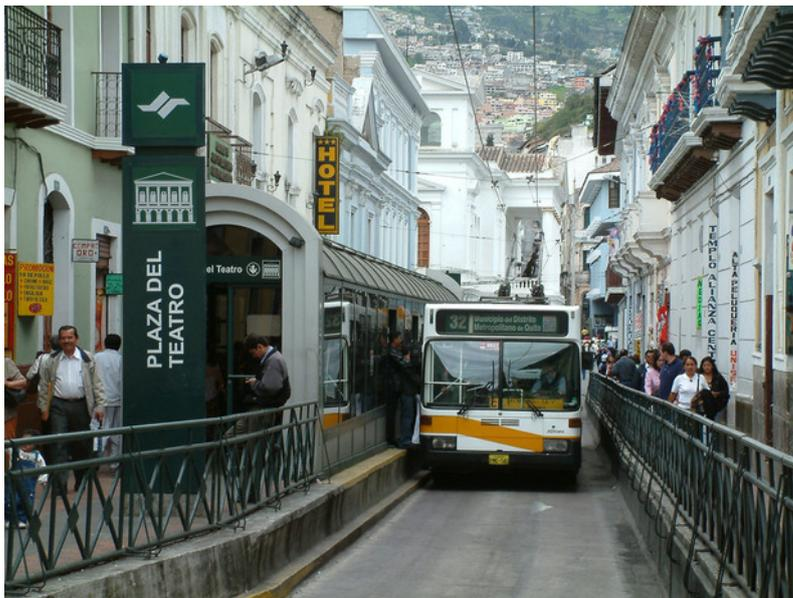
Figure 22.18. Insertion of bus lane and station in a narrow space in Quito. *Andre Frieslaar.*
