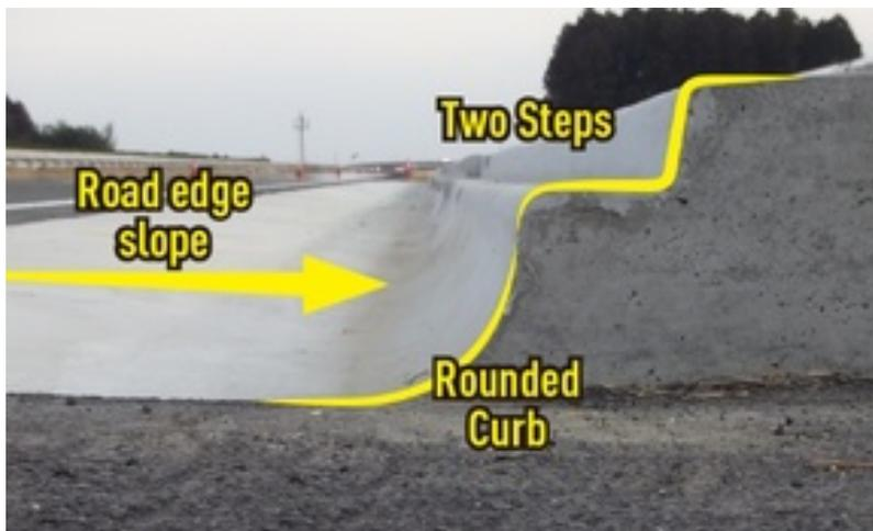
Figure 25.95. Image of the precision docking curb that shows the slope downward to the station, the rounded curb, and the idea of the stepping back the top of the curb. *Bridgestone*.
