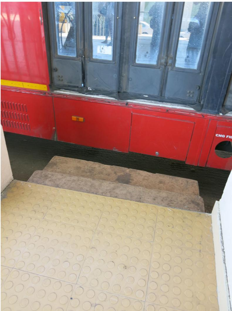
Figure 28.15. For customers transferring to and from the feeder buses that run in mixed traffic and are not high platform at Pimpri-Chinchwad's terminal, steps are built from the high platform of the station to the ground. ITDP
