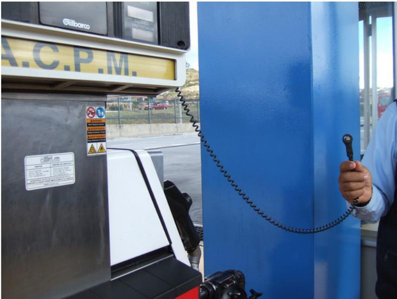
Figure 26.4. Upon entering the refueling area, a digital monitoring device records the pertinent vehicle details (i.e., fuel level, odometer, etc.). *Lloyd Wright.*
