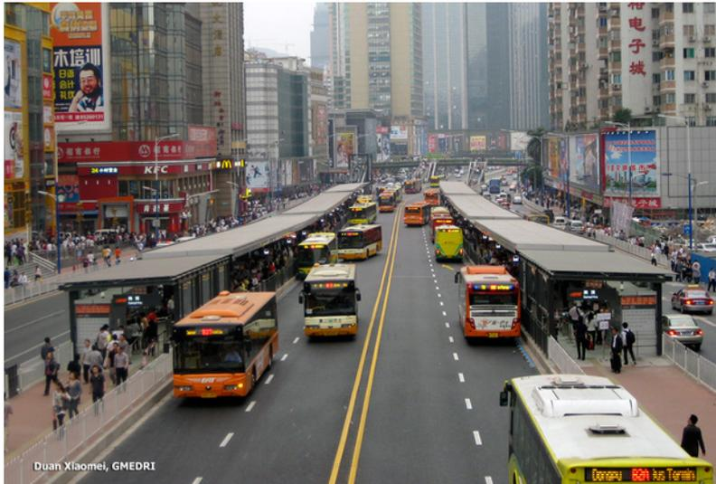
Figure 8.2. The Gangding BRT station in Guangzhou, China. Despite 24 meters being taken from the center of the roadway for the BRT stations and roadways, both capacity and speed of the road for mixed traffic and buses improved dramatically. Conditions for pedestrians were also greatly improved, with customers waiting in the station rather than on the side of the road. Duan Xiaomei, GMEDRI
