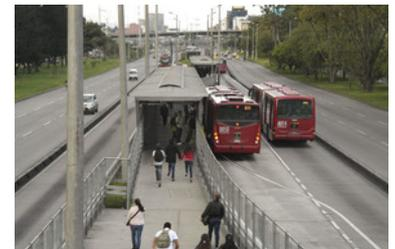
Figure 6.18. Passing lanes at stations, like these in Bogotá, allow for the provision of express and limited stop services. Karl Fjellstrom.
