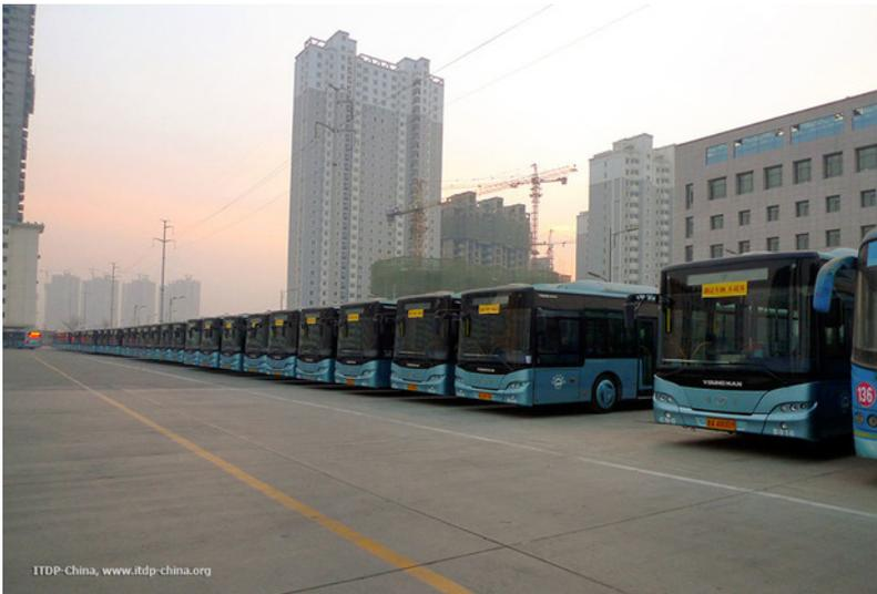
Figure 26.33. Use of concrete for bus parking areas and asphalt for bus circulation areas at a BRT vehicle depot the Lanzhou, China. Image *Karl Fjellstrom.*
