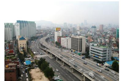
Figure 32.3. Before image of the Cheonggyecheon corridor project in Seoul, South Korea. Despite tearing down one of the principal expressways to the city, the resulting congestion impacts were minimal, especially since the new BRT corridors helped gain ridership from former car users. *Seoul Institute.*
