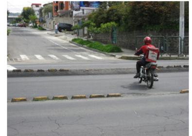
Figure 23.22. As more separator blocks erode, an increasing number of private vehicles intrude upon the busway, which can lead to serious accidents. Lloyd Wright
