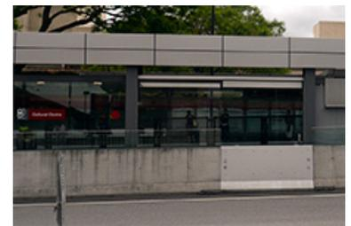
Figure 28.20. The noticeable differnet pannel is removable to provide additional access to a BRT station during high volume events such as New Year's Eve. Brisbane, Australia. *ITDP.*
