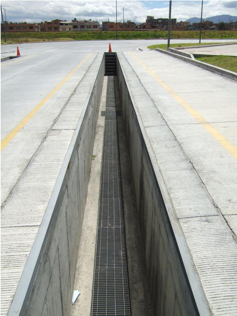
Figure 26.6. A channel allows the undersides of the vehicles to be washed *Lloyd Wright*
