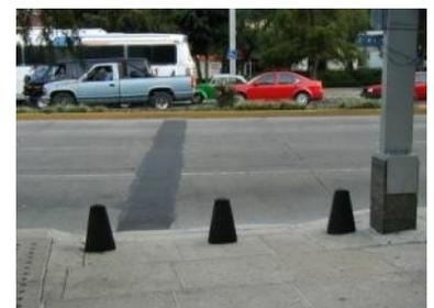
Figure 30.16. Curb ramps are required on both sides of the street, and at any median in between. The median opposite the curb ramp shown here in Mexico City lacks a curb ramp. Michael King.
