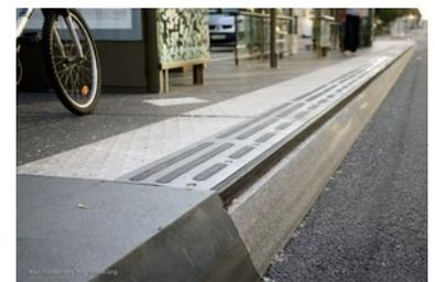
Figure 25.92. Smooth, hard, bevelled curb in Nantes to reduce tire wear. *Karl Fjellstrom*
