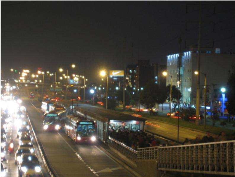
Figure 2.13. The provision of multiple stopping bays and passing lanes at stations permits the Bogotá TransMilenio system to achieve very high passenger capacities. *Carlos Pardo.*
