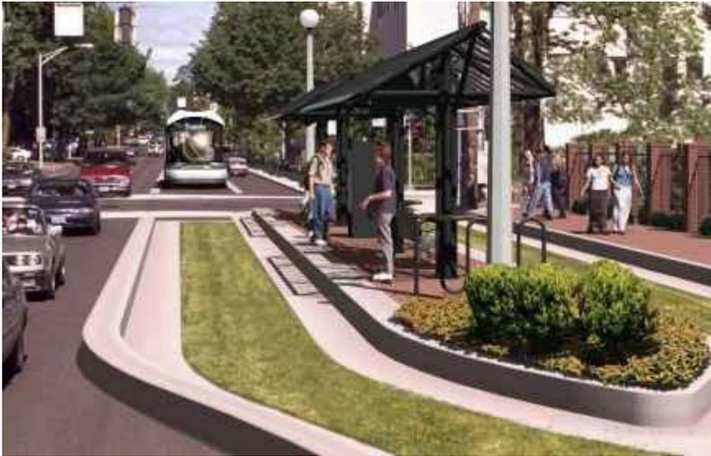
Figure 22.28. Not paving the center of the busway, like this example in Eugene, USA, may produce infrastructure cost savings as well as reduce operational noise. *Lane District Transit.*
