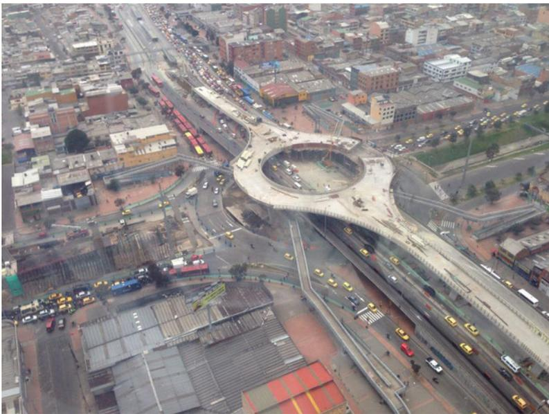
Figure 24.93. Exclusive BRT third-floor roundabout is an unprecedented work of art to guarantee free-flow movements for TransMilenio operation. *Instituto de Desarrollo Urbano de Bogotá*.
