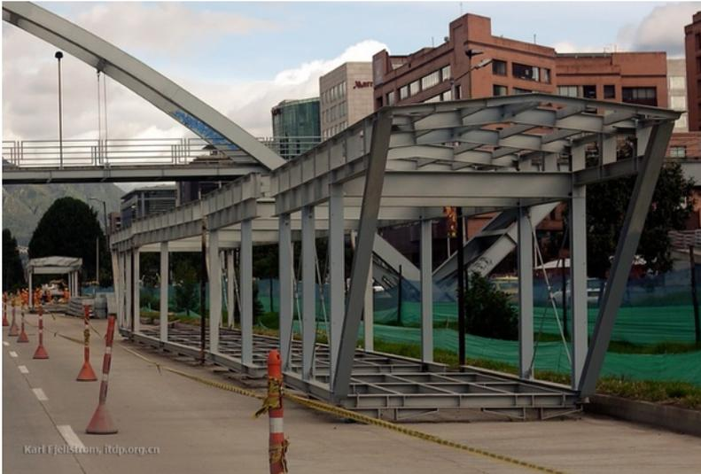
Figure 25.37. Prefabricated Bogotá BRT station module at the roadside, ready to be placed in position. *Karl Fjellstrom.*
