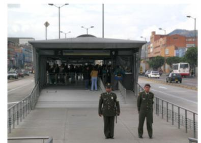
Figure 30.26. Ramp to BRT station, equal to the width of the station. *TransMilenio.*
