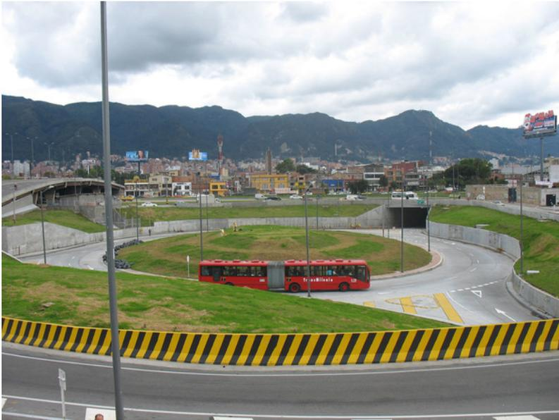
Figure 24.91. An exclusive roundabout facilitates exclusive turning movements for BRT vehicles between two corridors: the NQS corridor and Calle 80 corridor. *Eduardo Plata and Por el País que Queremos (PPO)*.
