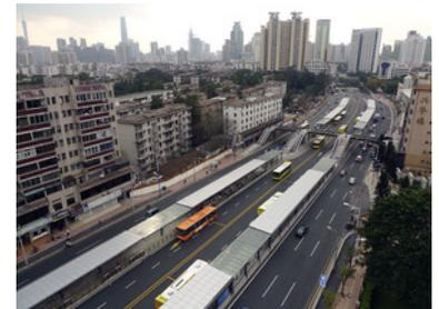
Figure 7.16. Shidajida BRT station in Guangzhou, at the midpoint underneath the access bridge, has one lane carrying 27,000 people and one vehicle every 10 seconds in a single direction during the peak hour. This system has the world's highest BRT vehicle carrying frequency. Image ITDP.
