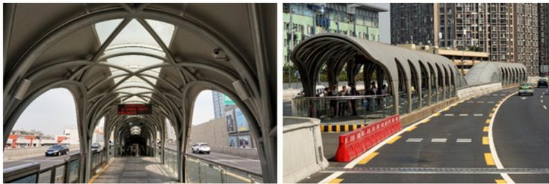
Figure 25.56. BRT station interior and exterior in Chengdu, which features stations with several different architectural styles. The skylight helps to ensure a bright interior and the walls curve downward. Karl Fjellstrom, ITDP
