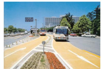
Figure 23.15. The coloration of busways does much to enhance the image and permanence of a BRT system. This photo shows a colorized busway in Nagoya, Japan. City of Nagoya
