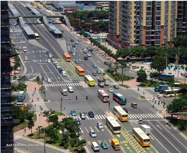
Figure 24.13. A typical major intersection on a BRT corridor in Guangzhou, China. Note that the station of the BRT corridor is located away from the intersection with Chibei Avenue, and in order to turn across traffic, the two-phase intersection requires a U-turn in the perpendicular road. Before the BRT, this four-phase intersection was a major traffic-congestion point. Image Karl Fjellstrom, ITDP.
