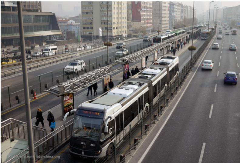
Figure 25.23. Medium-capacity station with high-capacity operation due to large buses, no defined stopping berths in Istanbul, Turkey. *Karl Fjellstrom.*
