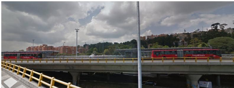
Figure 24.81. TransMilenio's Boyacá Station on the flyover is an example of adapting BRT to existing grade separation. *Google Street View.*
