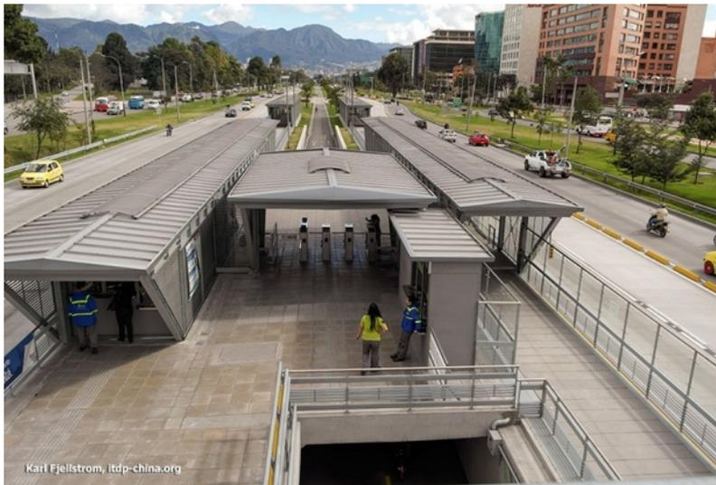
Figure 25.63. Straight row of turnstiles in a Bogotá BRT station with a segregated bike lane passing under the station. Karl Fjellstrom
