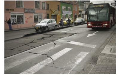
Figure 23.6. Damaged pavements along a TransMilenio corridor. Karl Fjellstrom, Far East BRT
