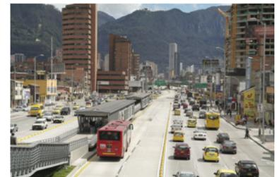
Figure 22.19. A median busway in Bogotá with a single median station has become the standard for high-quality BRT systems. ITDP.
