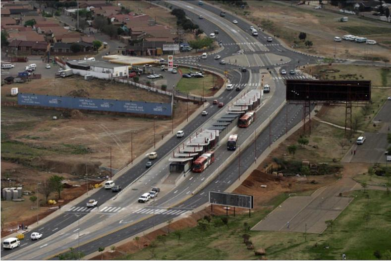
Figure 2.11. Rea Vaya in Johannesburg has two sub-stops, each with two docking bays, or the equivalent of four fully effective “loading bays,” able to board and alight passengers from sixteen doors simultaneously, something not considered in the TCQSM. *ITDP*.
