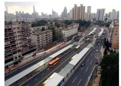
Figure 6.58. With only direct services in the Guangzhou BRT System, Shidajida station has four sub-stops and was designed with ample platforms and customer waiting space. Image Karl Fjellstrom, Far East BRT.
