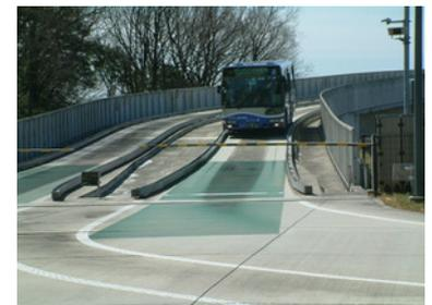
Figure 22.30. A stopping device at the end of the guideway ensures that the driver re-engages physical steering. *Lloyd Wright.*
