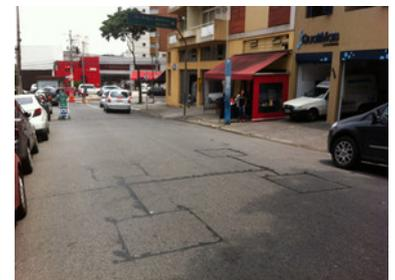
Figure 24.10. To feed São Paulo’s central traffic control, vehicles’ metallic surfaces are detected when approaching an intersection. *Arthur Szász.*
