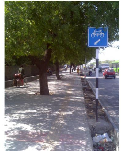
Figure 31.4. A protected bike lane—which provides physical separation from the roadway—along the BRT in Delhi, India, located between the roadway and trees. *Michael King.*
