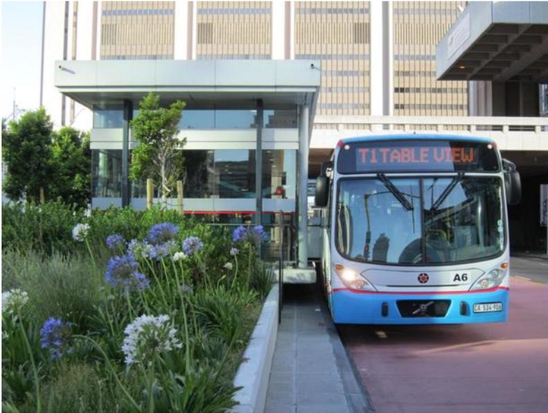
Figure 25.94. Cape Town uses Kassel curbs, a sloped curb that minimizes the wear and tear on the tires of the bus by curving up. *ITDP*
