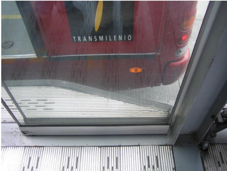
Figure 30.34. Sliding doors are a feature of many BRT systems. *TransMilenio*
