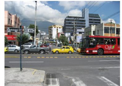
Figure 24.31. Prior to Quito's Ecovia line, mixed-traffic vehicles were allowed to cross through this intersection as well as negotiate cross-traffic and curbside turns. To give priority to public transport, crossing straight and cross-traffic turn movements have been blocked. *Lloyd Wright.*
