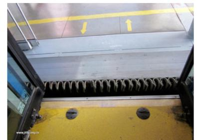
Figure 25.89. Cali's BRT stations feature padding to allow drivers to dock closely to the station. *Shanshan Li, ITDP*
