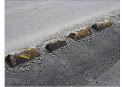
Figure 23.21. In Quito, the separator blocks have been susceptible to damage and deterioration. Lloyd Wright
