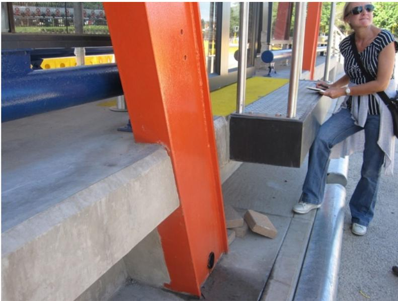
Figure 25.91. Pauline Froschauer standing next to Phase 1B construction of Johannesburg's BRT system. The curbs here are rounded and made of steel so that buses can pull up to them without damaging their tires. *Aimee Gauthier, ITDP*
