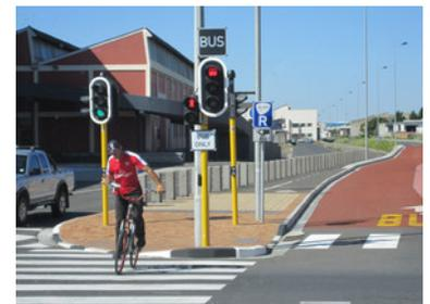
Figure 23.18. In Cape Town, South Africa, the separator between the busway and the mixed-traffic vehicles acts as a two-way bike lane and an island for pedestrians. *ITDP*
