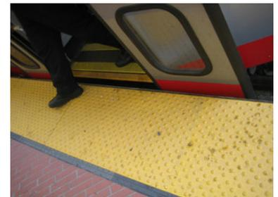
Figure 30.13. Warning strips mark platform edges of BRT and rail stations. Tom Rickert/AEI.
