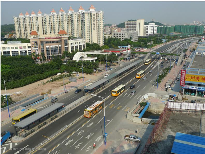
Figure 25.45. Two-sub-stop, offset split station in Guangzhou. The break in station roof coverage is due to the canal passing under the station at that point, and the access bridge has subsequently been covered. *ITDP.*
