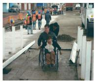
Figure 30.7. Mexico City's Metrobús invites disabled advisers to inspect stations during construction, in this case an access ramp. Secretaria de Obras y Servicios de México, DF,
