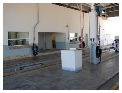
Figure 26.12. A pit beneath the work area allows technical staff to inspect (and service) the underside of the vehicle. Andre Frieslaar.
