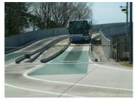
Figure 22.30. A stopping device at the end of the guideway ensures that the driver re-engages physical steering. *Lloyd Wright*.
