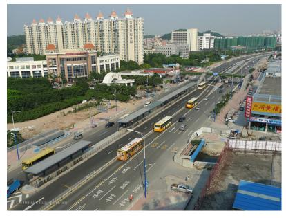
Figure 25.45. Two-sub-stop, offset split station in Guangzhou. The break in station roof coverage is due to the canal passing under the station at that point, and the access bridge has subsequently been covered. *ITDP*.
