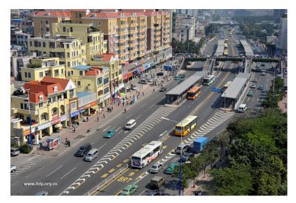
Figure 24.21. Double to single BRT lane transition before intersection in Guangzhou, China. Karl Fjellstrom, ITDP.
