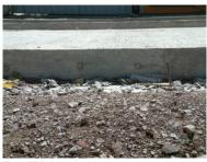
Figure 23.7. Reinforced concrete, as in this example from the construction of the Quito Central Norte line, has much greater longevity than asphalt. *Lloyd Wright*
