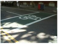
Figure 24.72. In the UK, a priority bicycle stopping area is placed ahead of the stopping line for motorized vehicles. *Lloyd Wright*.
