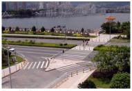
**Figure 29.25.** A median in the center of the road keeps drivers from swinging wide during a turn in Shenzhen, China. *Karl Fjellstrom, Far East BRT*
