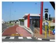
Figure 23.17. Colorized concrete adjacent to epoxycoated asphalt on Cape Town's MyCITI system. Andre Frieslaar
