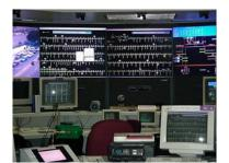
Figure 27.8. A large-screen display and vehicle tracking board can help staff and supervisors quickly assess the situation. Los Angeles County Metropolitan Transportation Authority.
