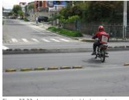
Figure 23.22. As more separator blocks erode, an increasing number of private vehicles intrude upor the busway, which can lead to serious accidents. Lloyd Wright
