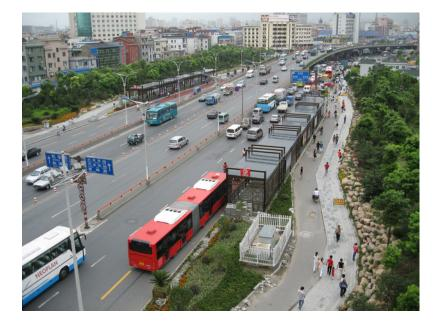
Figure 31.14. The bike lane along the Hangzhou, China, BRT system is sited between the BRT lane and the sidewalk. Karl Fjellstrom.
