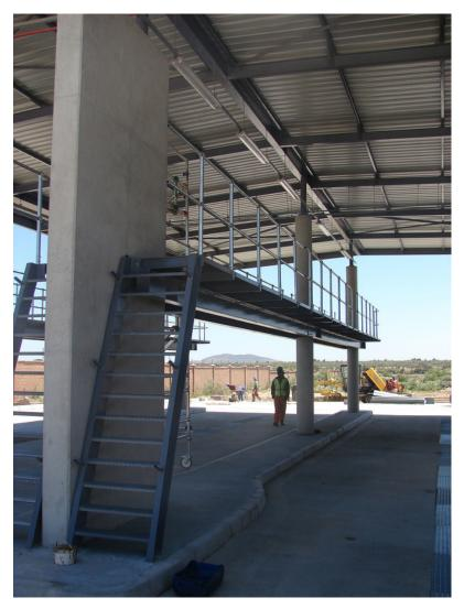
Figure 26.9. Stairs and a catwalk give access to the vehicle roof for washing purposes. Andre Frieslaar.
