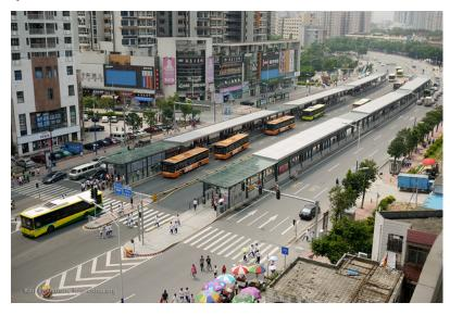
Figure 25.13. Dongpu BRT station in Guangzhou shows the station divisions including the access and arrival areas, the entrance area including the space for fare collection, and the three sub-stops, which can be identified by the different roof material and variation in elevation. At each sub-stop, multiple docking bays are seen and the station includes passing lanes. Between sub-stops is space for buses to pull into or out of the station around other buses already docked. *Karl Fjellstrom*.
