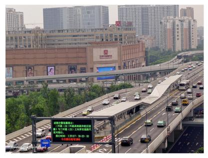
Figure 25.44. Offset central station in Chengdu without passing lanes or sub-stops. Xianyuan Zhu, ITDP.
