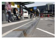
Figure 25.93. Smooth, hard, bevelled curb in Amsterdam to reduce tire wear. *Karl Fjellstrom*
