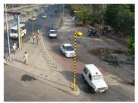
Figure 29.27. A raised crosswalk on the Delhi, India, busway helps reduce the speed of left-turning vehicles. *Chris Kost*
