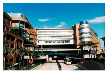
Figure 22.33. An exclusive busway runs under the Mater Hill Hospital in Brisbane. Queensland Transport.
