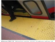
Figure 30.13. Warning strips mark platform edges of BRT and rail stations. *Tom Rickert/AEI*.
