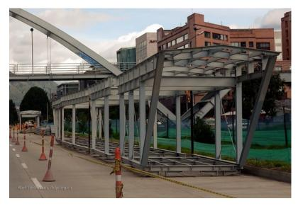
Figure 25.37. Prefabricated Bogotá BRT station module at the roadside, ready to be placed in position. Karl Fjellstrom.
