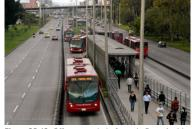
Figure 25.42. Offset central platforms in Bogotá witi passing lanes and sub-stops. *Karl Fjellstrom*.
