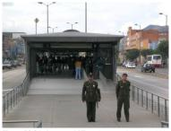
Figure 30.26. Ramp to BRT station, equal to the width of the station. *TransMilenio*.
