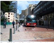
Figure 23.8. Bogotá's TransMilenio resurfaced the entire corridor in concrete and used brick in the city center for aesthetic reasons. *Carlosfelipe Pardo*
