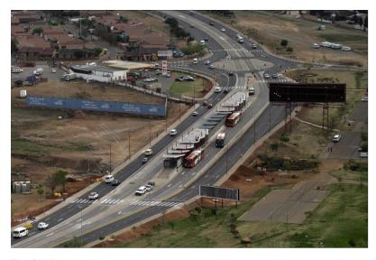
Figure 2.11. Rea Vaya in Johannesburg has two sub-stops, each with two docking bays, or the equivalent of four fully effective "loading bays," able to board and alight passengers from sixteen doors simultaneously, something not considered in the TCQSM. *ITDP*.
