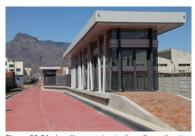
Figure 22.56. An off-set station in Cape Town, South Africa. The platforms are arranged a distance apart to allow for a passing lane on each side at the station docking area. *ITDP*.
