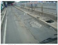
Figure 23.9. TransJakarta, in Jakarta, Indonesia, initially used only asphalt and suffered from major problems of the roadway sinking and deteriorating at the stations, so the roadbed at the stations was repaved using concrete. *ITDP*
