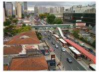
Figure 16.4. São Paulo's Passa Rapido corridors had severe station saturation problems until reconstructed. BRT Planning International, LLC.
