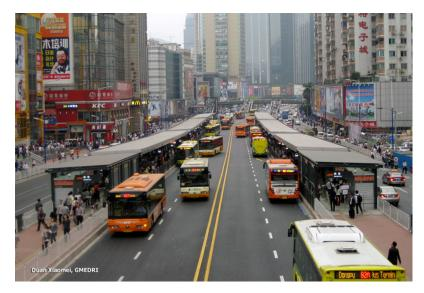
Figure 8.2. The Gangding BRT station in Guangzhou, China, Despite 24 meters being taken from the center of the roadway for the BRT stations and roadways, both capacity and speed of the road for mixed traffic and buses im proved dramatically. Conditions for pedestrians were also greatly improved, with customers waiting in the station rather than on the side of the road. Duan Xiaomei, GMEDRI
