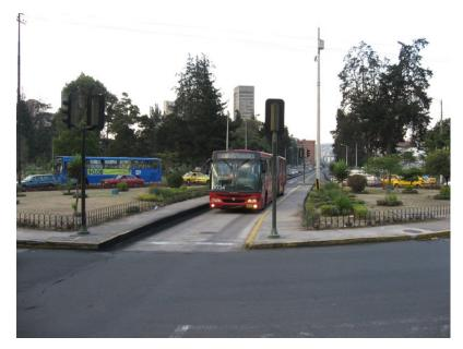
Figure 24.67. Quito's Ecovía line cuts directly through a roundabout. Lloyd Wright.
