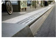
Figure 25.92. Smooth, hard, bevelled curb in Nantes to reduce tire wear. *Karl Fjellstrom*
