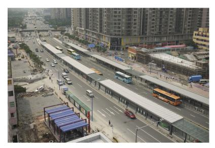
Figure 22.60. A multiple sub-stop, split, side-aligned station in Guangzhou, China. ITDP.
