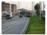
Figure 23.20. In Bogotá, the separator blocks are high enough to discourage intrusions by private vehicles but low enough to allow a BRT vehicle to leave the busway in case of emergency. *Carlosfelipe Pardo*
