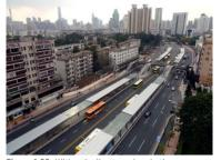
Figure 6.58. With only direct services in the Guangzhou BRT System, Shidajida station has four sub-stops and was designed with ample platforms and customer waiting space. Image Karl Fjellstrom, Far East BRT.
