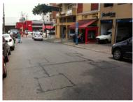
**Figure 24.10.** To feed São Paulo's central traffic control, vehicles' metallic surfaces are detected when approaching an intersection. *Arthur Szász*.
