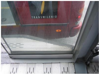
Figure 30.34. Sliding doors are a feature of many BRT systems. TransMilenio
