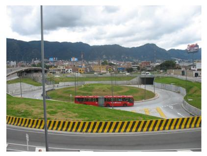
Figure 24.91. An exclusive roundabout facilitates exclusive turning movements for BRT vehicles between two corridors: the NQS corridor and Calle 80 corridor. Eduardo Plata and Por el País que Queremos (PPQ).
