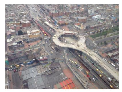
Figure 24.93. Exclusive BRT third-floor roundabout is an unprecedented work of art to guarantee free-flow movements for TransMilenio operation. Instituto de Desarollo Urbano de Bogotá.
