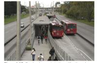
Figure 6.18. Passing lanes at stations, like these in Bogotá, allow for the provision of express and limited stop services. *Karl Fiellstrom*.
