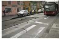
Figure 23.6. Damaged pavements along a TransMile nio corridor. Karl Fiellstrom. Far Fast BRT
