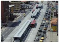
Figure 7.15. The use of multiple sub-stops, in this case three in each direction, has been one of the principal reasons Bogotå is able to achieve very high customer capacities. Photo Akiris.
