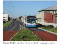
Figure 23.12. Section of colored friction course with ultrathin asphalt on Cape Town's MyCITI system. Aimee Gauthier
