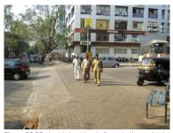
Figure 29.23. At this junction in Pune, India, a raised pedestrian crossing compels drivers to slow down and allows pedestrians to remain at the same level while crossing to the other side. *Chris Kost*
