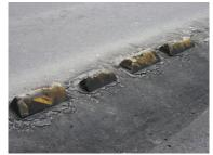
Figure 23.21. In Quito, the separator blocks have n susceptible to damage and deterioration. Lloyd
