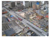
Figure 6.8. The use of multiple sub-stops and docking bays with passing lanes in Bogotá helps minimize vehicle congestion. Oscar Diaz and Por el País que Queremos (PPQ).
