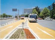
Figure 23.15. The coloration of busways does much to enhance the image and permanence of a BRT system. This photo shows a colorized busway in Nagoya Japan. *City of Nagoya*
